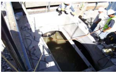
Manhole construction for the Spanish Springs Interceptor
