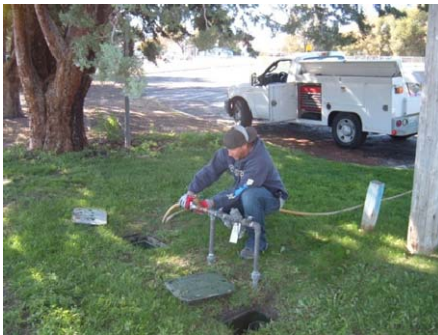
Brandon Miles Winterizing the irrigation system near Oddie and Pyramid
