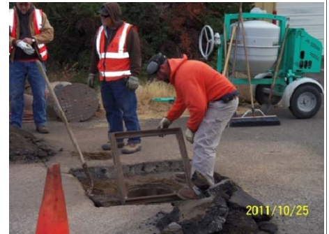
Clint Larson, Bo Collins, and Jeff Parmenter raising a manhole on Dermody Way.
